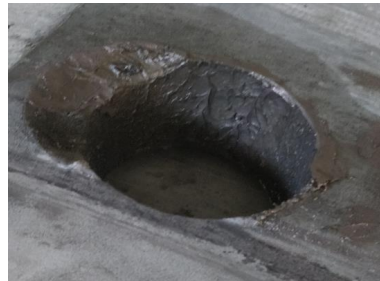
Rotor lock repair
