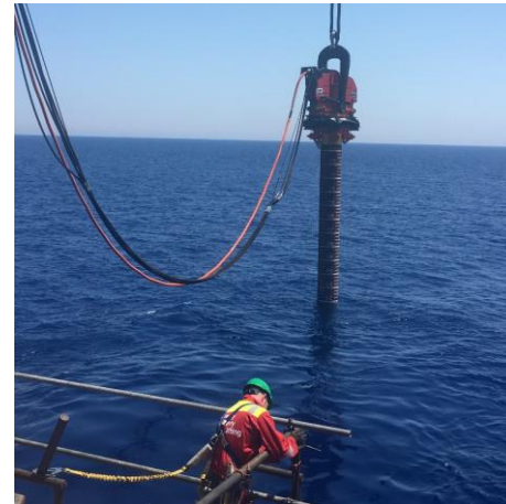
PIN/JACKET PILE INSTALLATION
