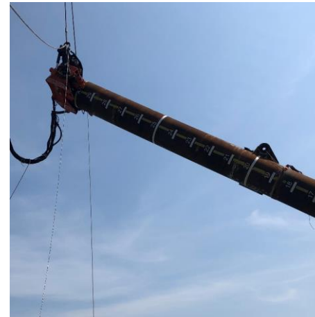
ANCHOR PILE INSTALLATION
