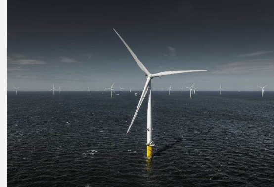
Monopile (Burbo Bank Extension)
